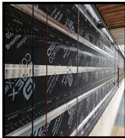
Elevation 3 -Top hat - breather membrane installation
