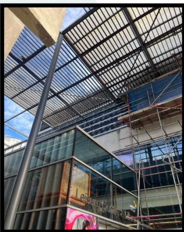
Elevation 3 -Top hat - breather membrane installation
