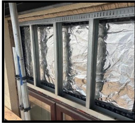
Picture's showing the SFS and EPDM, installed to phase 1
