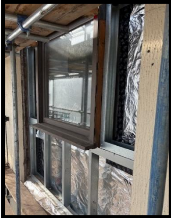
Picture's showing the SFS and EPDM, installed to phase 1
