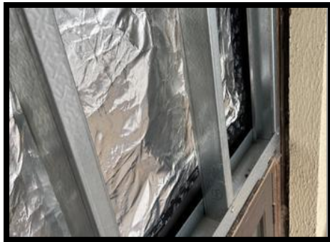
Pictures showing - 70% of EPDM, insulation, metal stud board and breather membrane on phase 1&2
