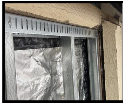
Pictures showing - 70% of EPDM, insulation, metal stud board and breather membrane on phase 1&2
