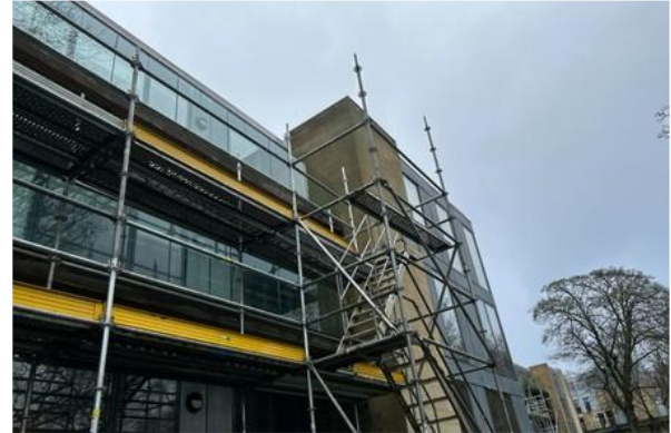
Bluebell House Scaffold
