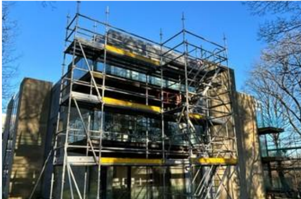
Bluebell House Scaffold
