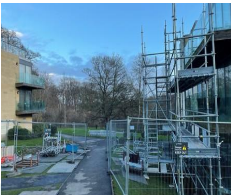
Bluebell House Scaffold
