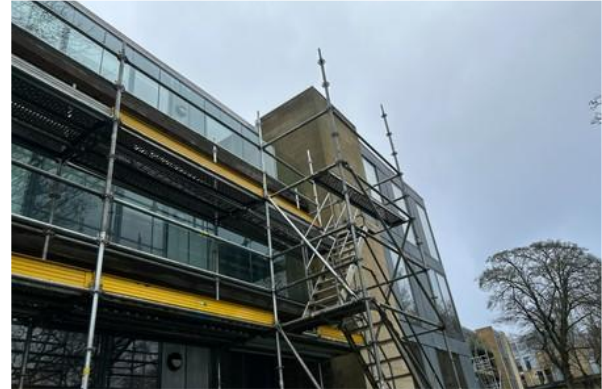
Bluebell House Scaffold
