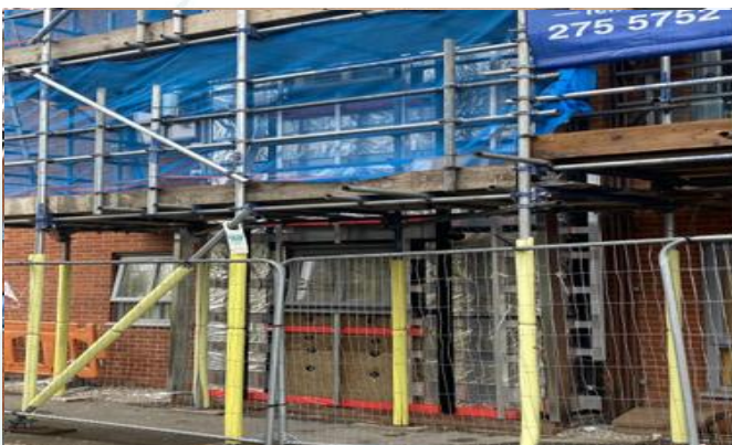
Photo Showing Progression On C1 Channels, Brackets, Rails & Fire Barrier
