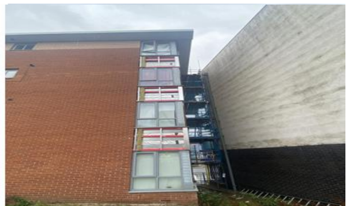
A Photo Showing Area Now Ready For Insulation
