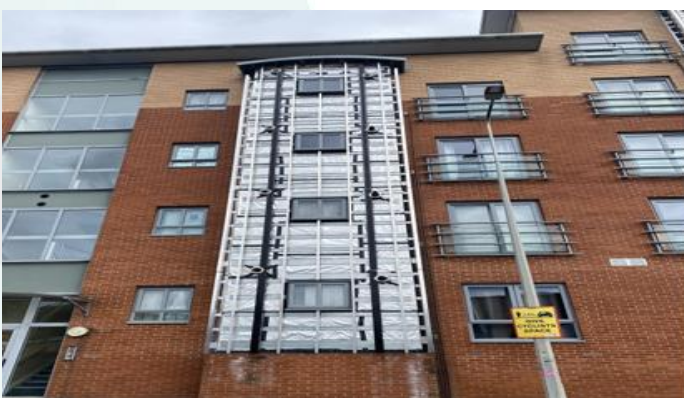
B1 Now Ready For Fire Stop & Insulation
