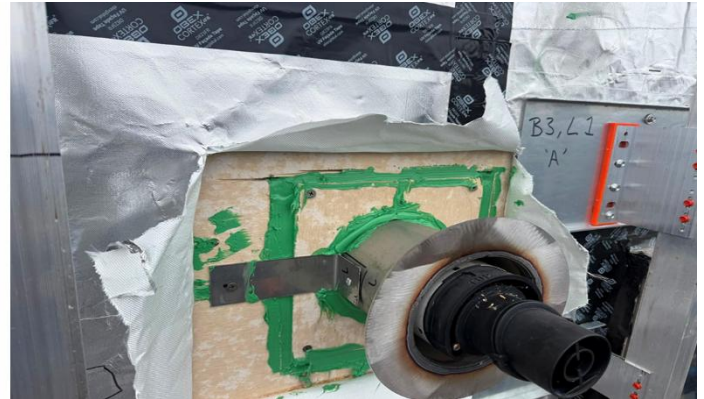
Close Up Photo Of The Installation Of The Stainless Steel Boiler Tubes
