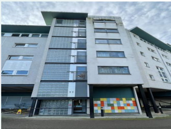
Blockwork removal phase 2
