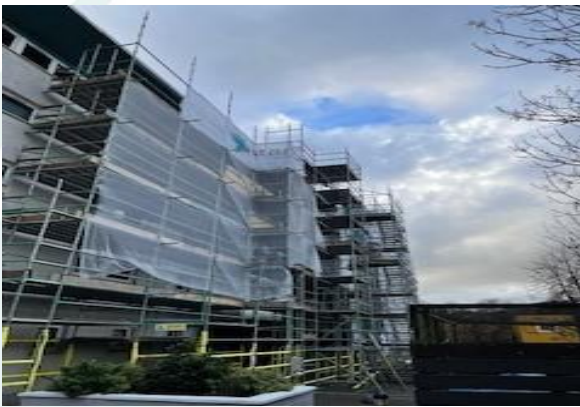
Phase 2 scaffolding ongoing
