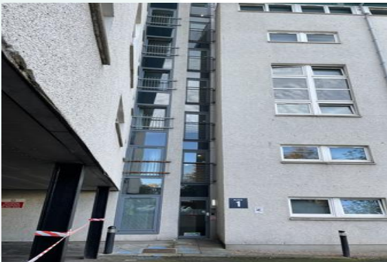
Blockwork Removal Block 1
