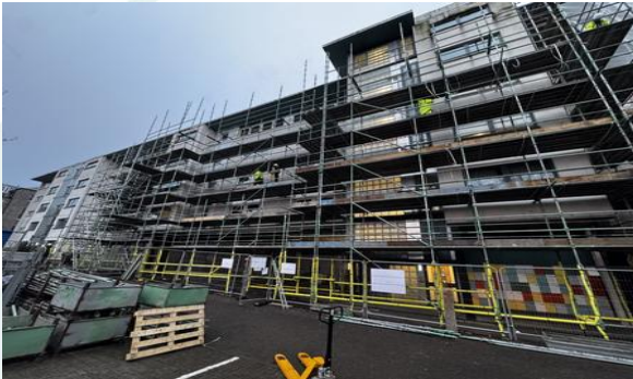
Phase 2 scaffolding ongoing
