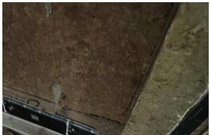
A photo showing Phase North Elevation – Knauf Rocksilk Insulation installation works to staircase concrete shear wall progressing.
