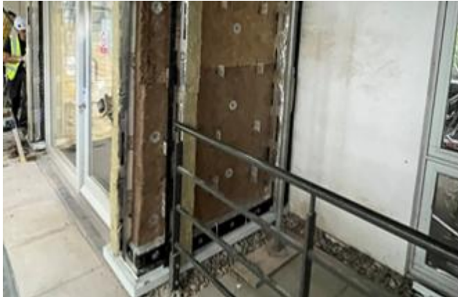
A photo showing Phase North Elevation – Cavity Fire Barrier installation works to staircase concrete shear wall progressing.
