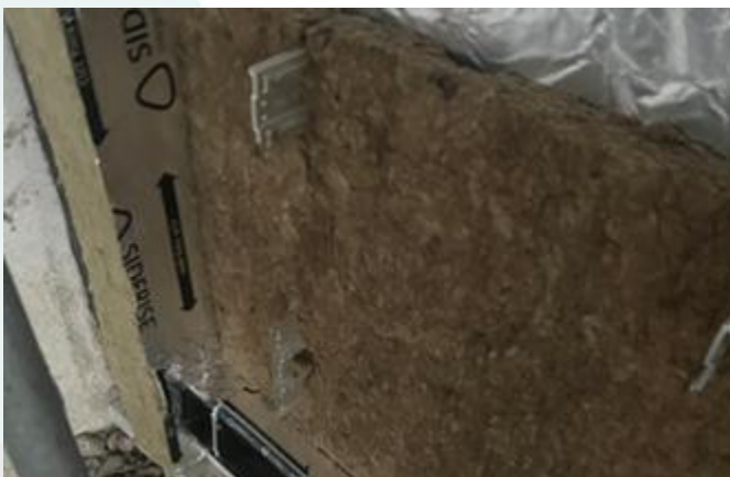
A photo showing Phase North Elevation – Knauf Rocksilk Insulation installation works to staircase concrete shear wall progressing.
