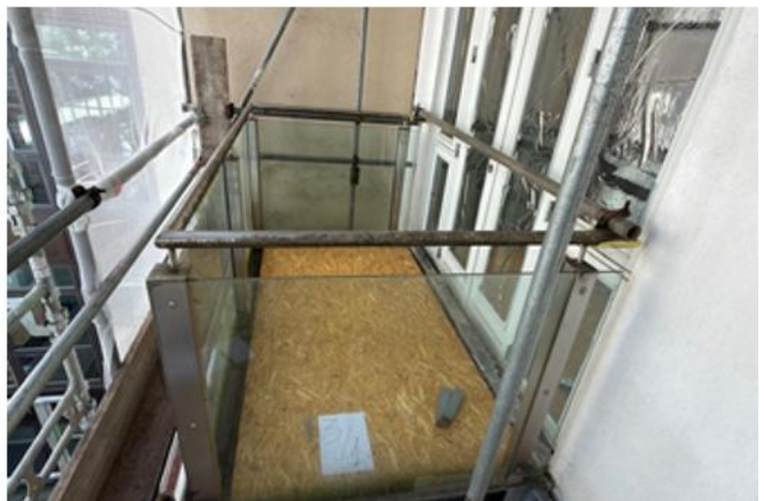
A photo showing Phase 2 North Elevation – Existing decking replacement works complete and temporary protection in place
