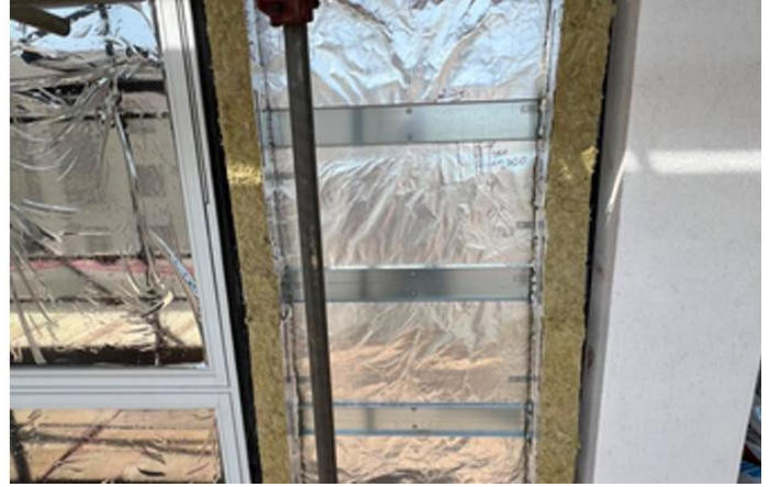
A photo showing Phase 1 South Elevation – Siderise cavity fire barriers installation works commenced.
