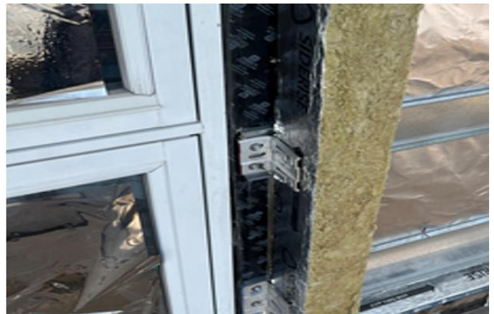
A photo showing Phase 1 South Elevation – Helping hand bracket installation works commenced
