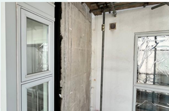
A photo showing Phase 2 North Elevation – Existing cladding removal works progressing
