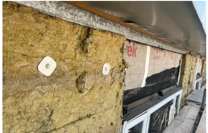
A photo showing Phase 2 North Elevation – Existing cladding removal works progressing
