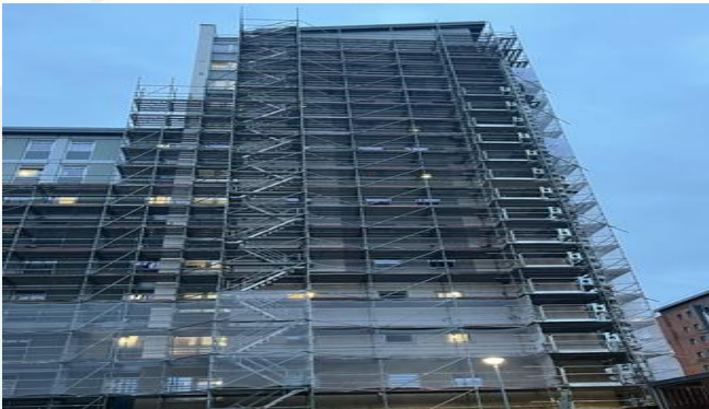
phase 1 scaffolding ongoing
