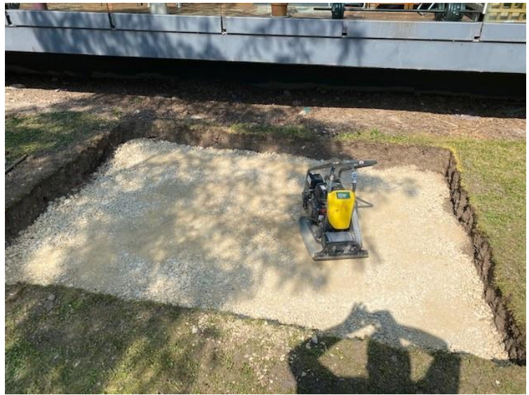
Block 2 – Excavation of soft landscape areas
