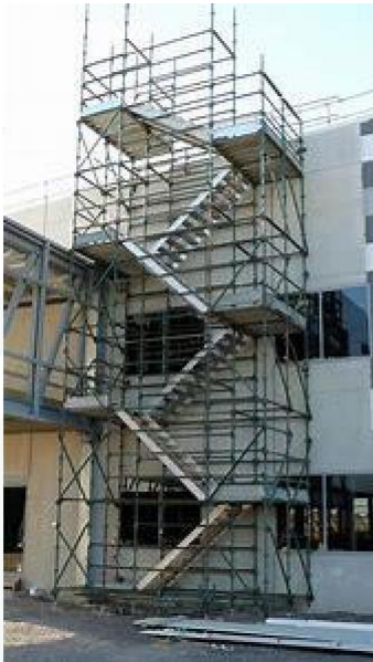
An example of a haki staircase.
