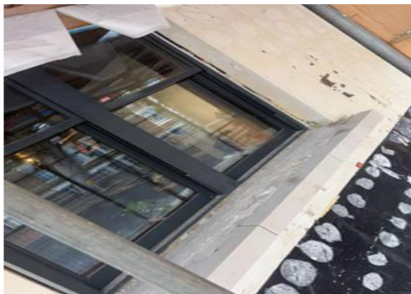
A photo Showing Render Removal
