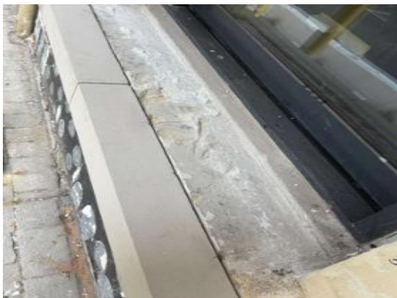
A photo Replacements of New Stone Cills ongoing
